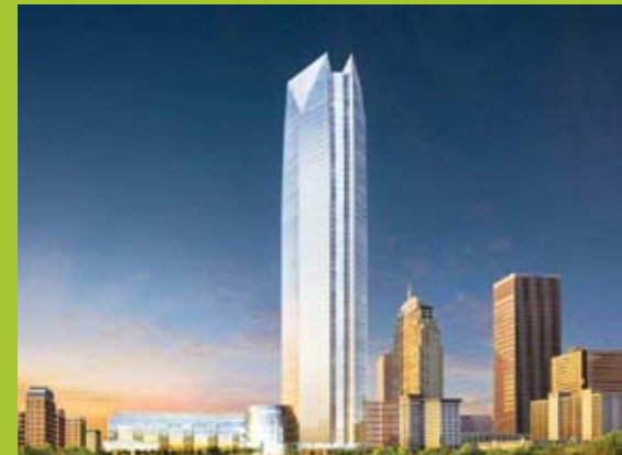
The new world headquarters for Devon Energy scrapes the sky above Oklahoma City, Oklahoma. Atlas agents Alexander's Mobility Services and Ace Moving & Storage partnered to provide the consolidation and relocation of offices for 2300 employees here. The massive project unfolded in sixteen phases between March and October and entailed the transport of 600 truckloads. "The Alexander's team was excellent to work with," says President Ernie Dean, Ace Commercial Moving & Storage (1408). "Their experience and leadership made a big difference."
