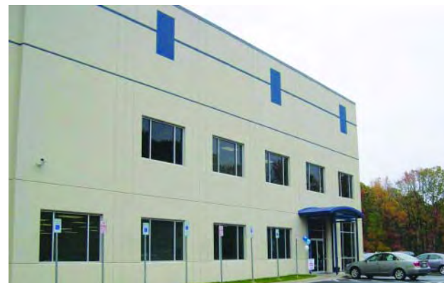
The newest Alexander's Mobility Services facility houses offices and warehouse in the "Crossroads@95" business park east of Baltimore. The company held an open house in November to showcase the 130,000 sq. ft. custom building. It features 118,000 sq. ft. of warehouse space and a state-of-the-art system for inventory control.
